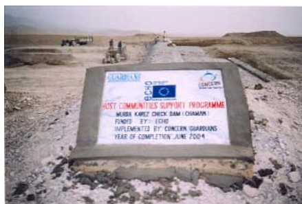
Check Dam Murda Karez
